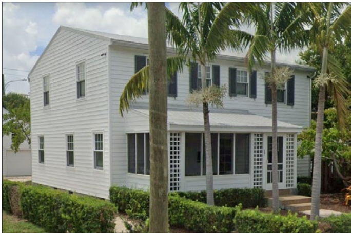
Figure 24 This image is of the beautifully restored 14 South “M” Street structure which currently houses the city’s Leisure Services Dept.
